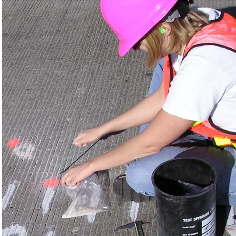
FIGURE 3.10 Concrete sampling for chloride concentration analysis.
