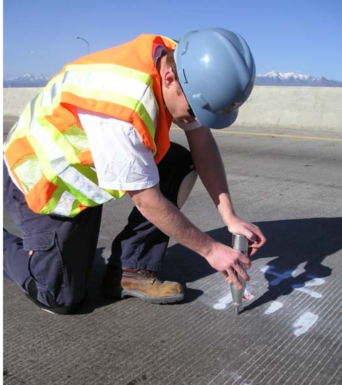
FIGURE 3.7 Schmidt hammer rebound testing.
